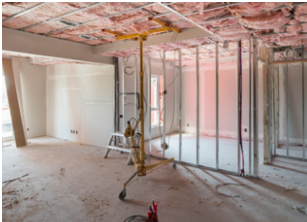
Suspended-ceiling cavities are filled with mineral soundproofing wool © Photo: Stéphane Groleau
