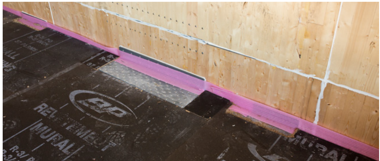
Acoustic seal between CLT panels and soundproofing membrane on the floor © Photo: Stéphane Groleau
