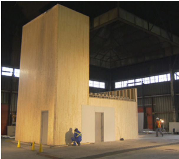
Assembly for the full scale fire demonstration test © Photo: Nordic Structures
