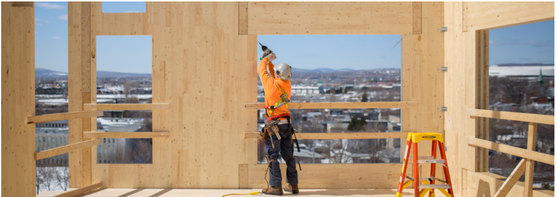
The wall panel rises above the floor level, doubling as a guard rail
