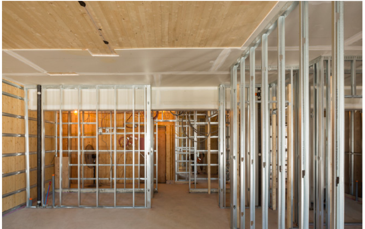
Metal frame to reduce the combustible load © Photo: Stéphane Groleau
