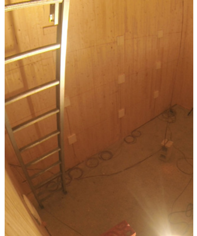
Stairs/elevator shaft at the end of the large scale demonstration test © Photo: Nordic Structures
