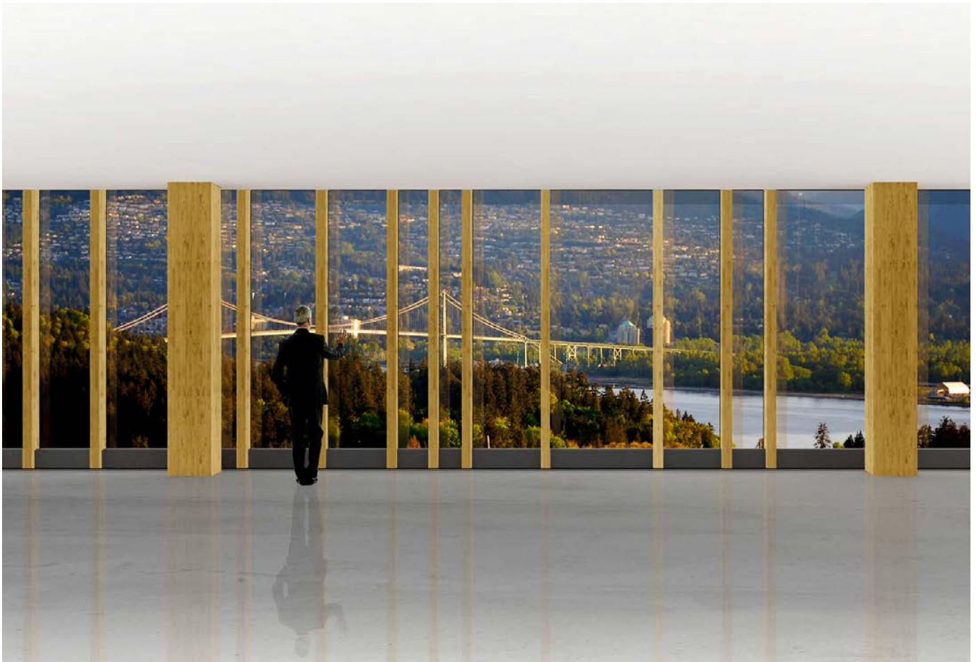
Interior perspective illustrating a glulam curtain wall
