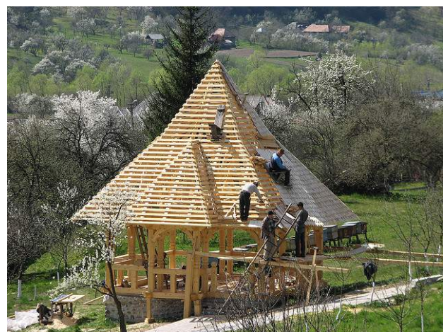
One of the smaller churches under repair showing the type of wood construction used in all of the monastery structures.
