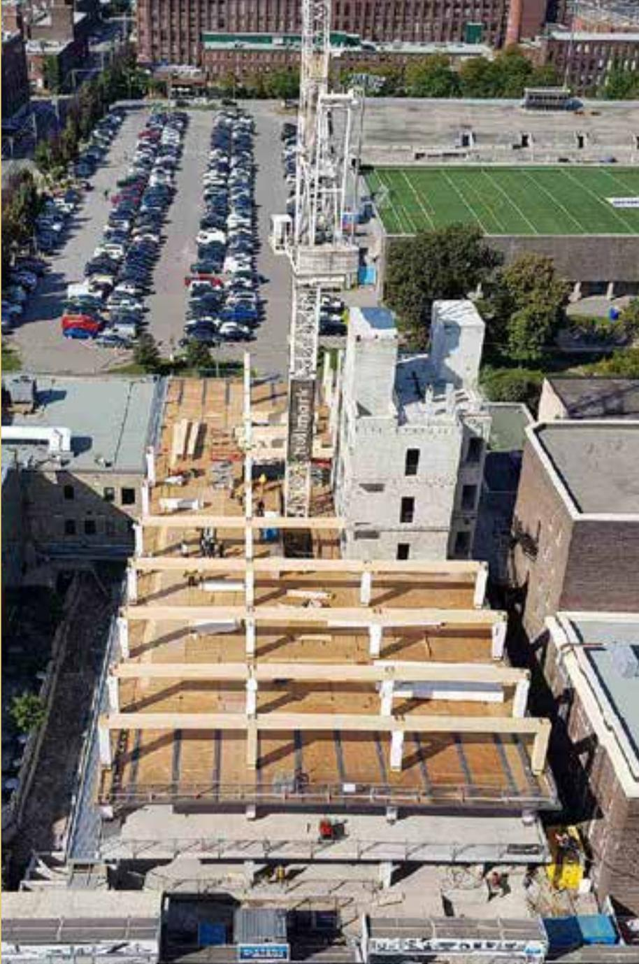
**Bird's-eye view of 80 Atlantic during the installation of the timber columns and beams for the third floor.**
