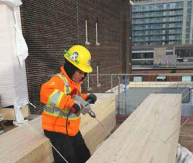
Carpenter uses 600 mm screws to stitch together two pieces of glulam to complete the assembly of a beam prior to its installation.
