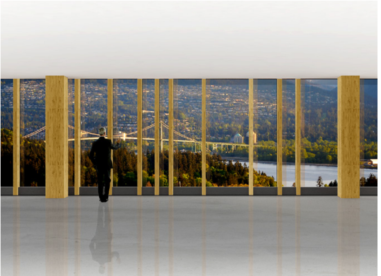
Interior perspective illustrating a glulam curtain wall
