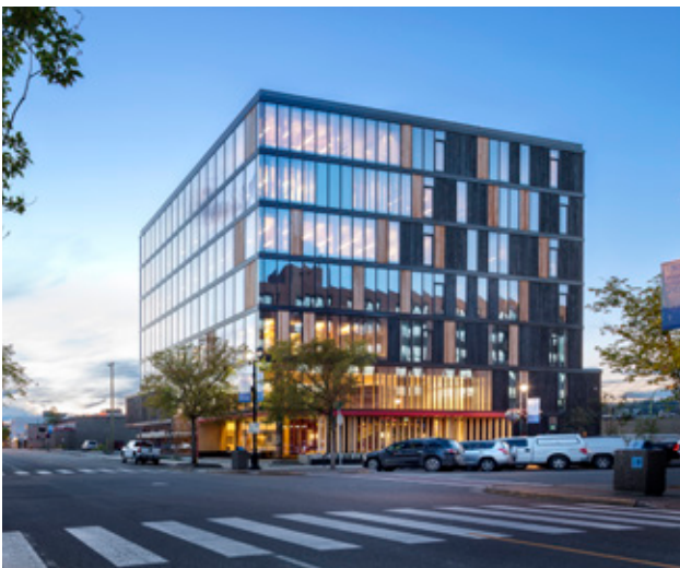
ADDENDA: WOOD INNOVATION AND DESIGN CENTRE: A CASE STUDY IN BRITISH COLUMBIA. IMAGE: MICHAEL GREEN ARCHITECTURE
