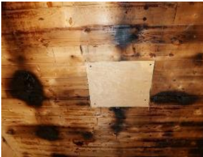
c) Test 1-2 CLT repaired with plywood
