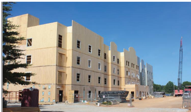
Figure 18. Redstone Arsenal hotel under construction (photo credit LendLease) [77]
