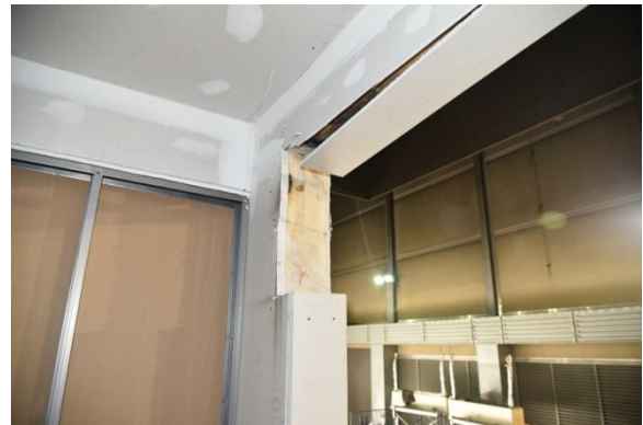
f) charred section removed at window
