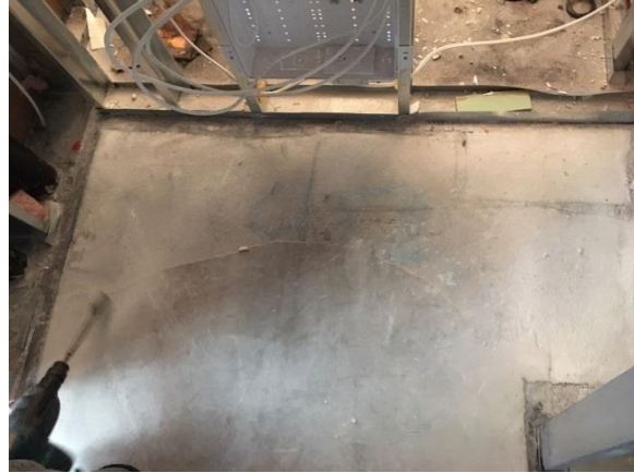
b) Condition of slab after water removal
