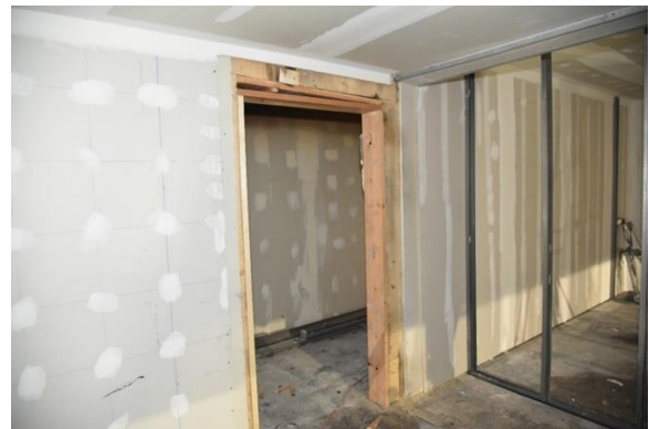
h) repaired apartment door frame
