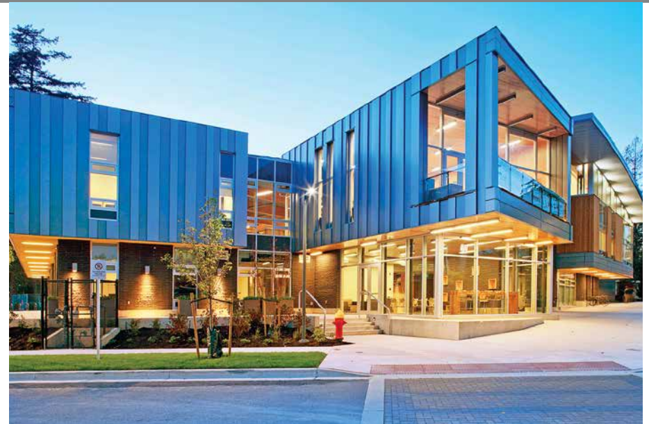
2.2 Wesbrook Community Centre gymnasium
