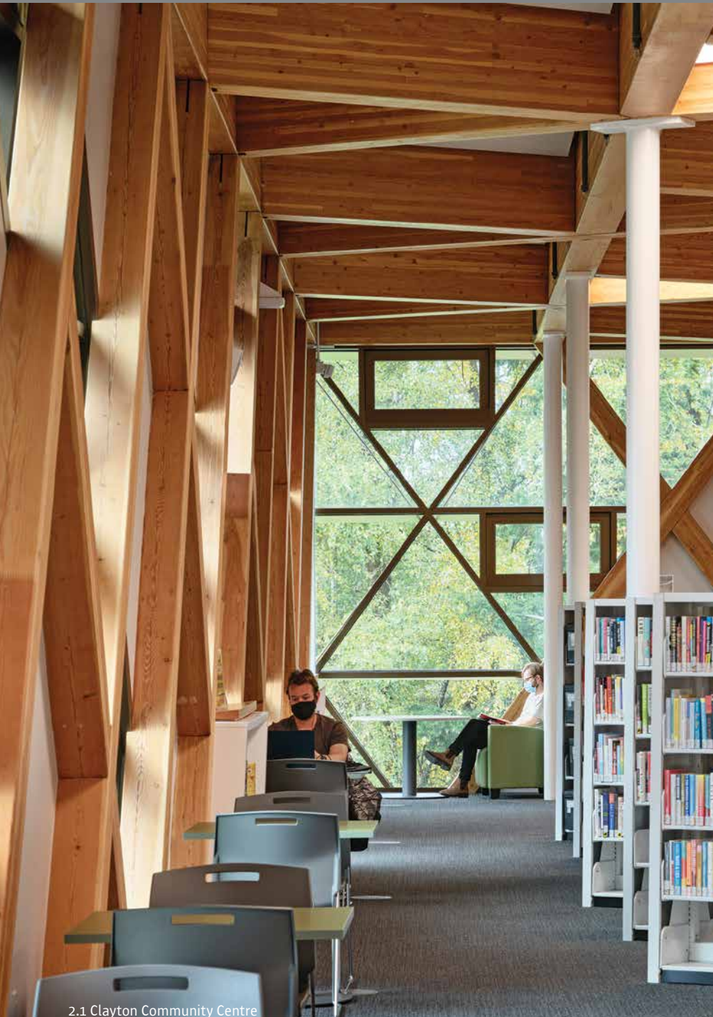
2.1 Clayton Community Centre
