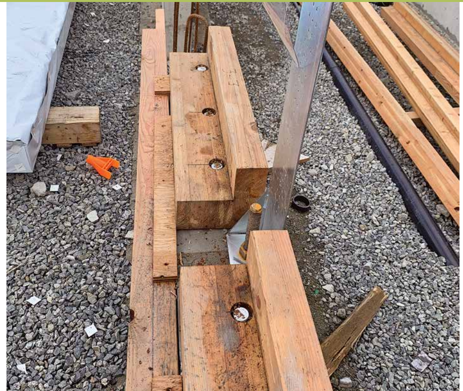
5.15 Glulam ledger detail at concrete upstand
