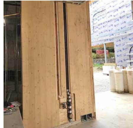
6.8 A chase routed into the CLT to conceal conduit
