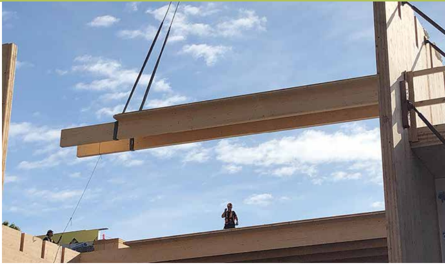
5.13 Double Tee installation
