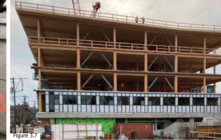
Figure 3.5 and 3.6: Installing a raised floor helped conceal building services, with the void acting as a plenum for air distribution. (Credit DBS) Figure 3.7: The optimal structural system was based on a 6.1m x 6.1m grid, with beams in one direction only and the CLT panels spanning across two bays. (Credit Aspect Structural Engineers) Figure 3.8: 3.8 CLT to glulam beam connection at panel junction. (Credit Aspect Structural Engineers) Figure 3.9: CLT to glulam beam connection mid-panel. (Credit Aspect Structural Engineers)
